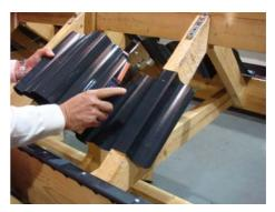
6. Fix the tray onto the rafters using corrosion resistant clout head nails or staples.
