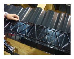
11. Adjoining lengths should be overlapped by a minimum of 100mm. Lay the roofing underlay onto the Underlay Support Tray, ensuring the bottom edge does not go over the line of the fascia board and into the gutters.
