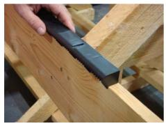
1. Position the Fascia Vents directly on top of the fascia board with the stop section firmly against the vertical edge of the fascia board.
