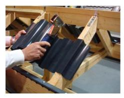
5. Roll out the Roll Out Rafter Tray over the rafters in the correct position to provide a clear ventilation channel above the roof insulation.
