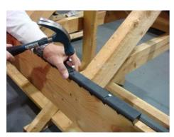
3. Fix the Fascia Vents onto the top of the fascia board through the nail holes using 50mm x 3.35mm corrosion resistant nails.
