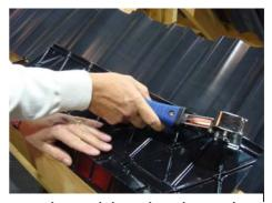
10. Then nail them directly into the rafters using corrosion resistant nails or staples.
